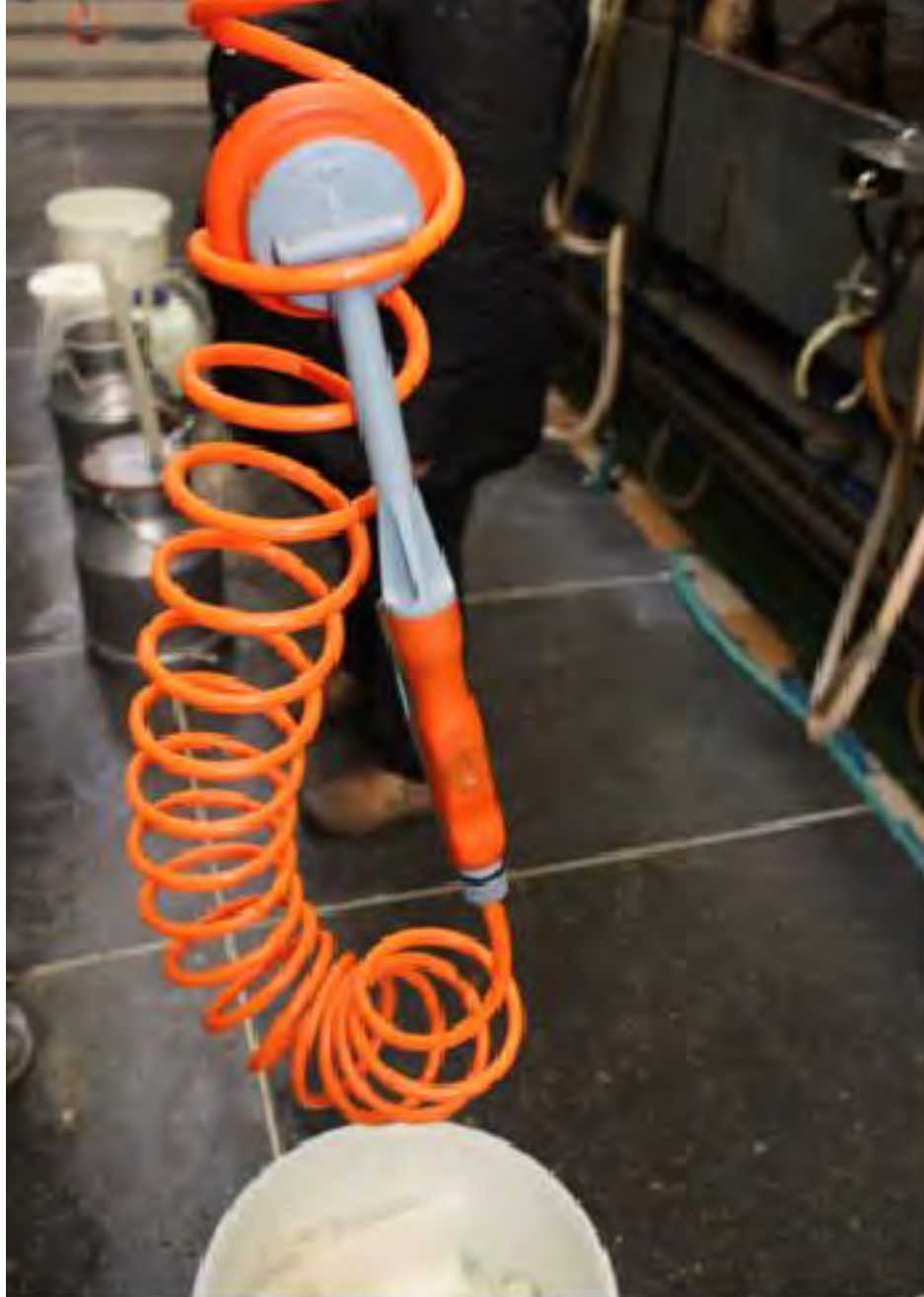
Mirošov - spray system
